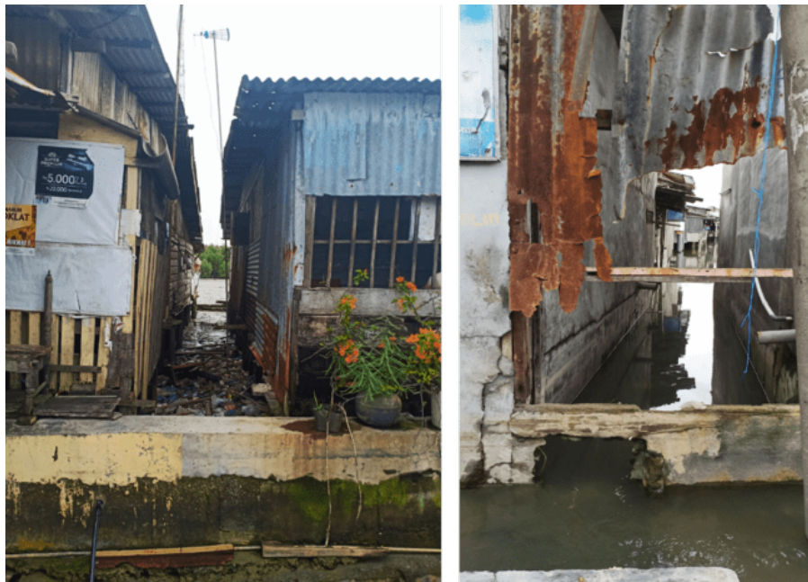
Picture 1-4 Damage to building materials due to flooding
